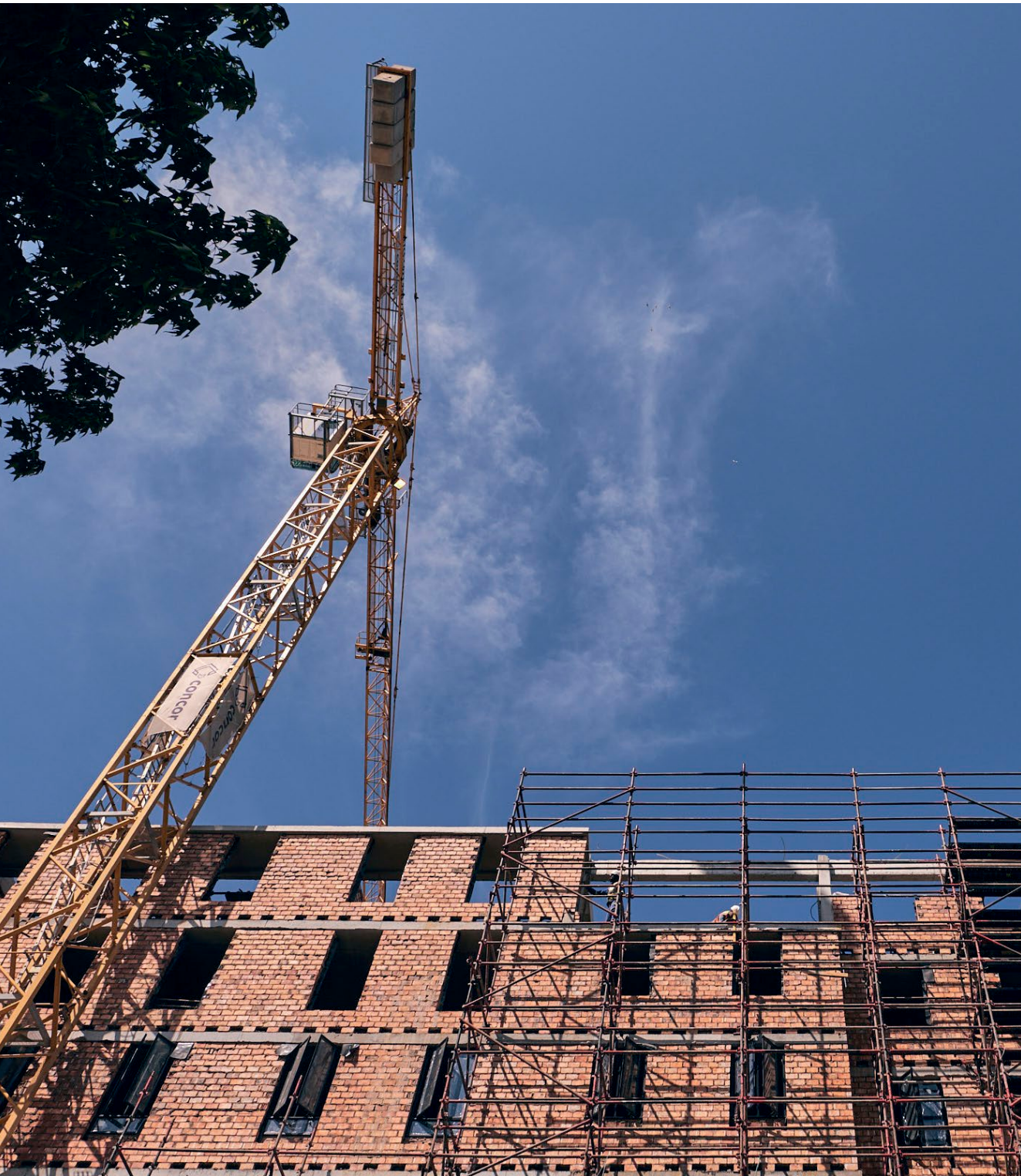
Student accomodation underway in Main Road, Claremont
