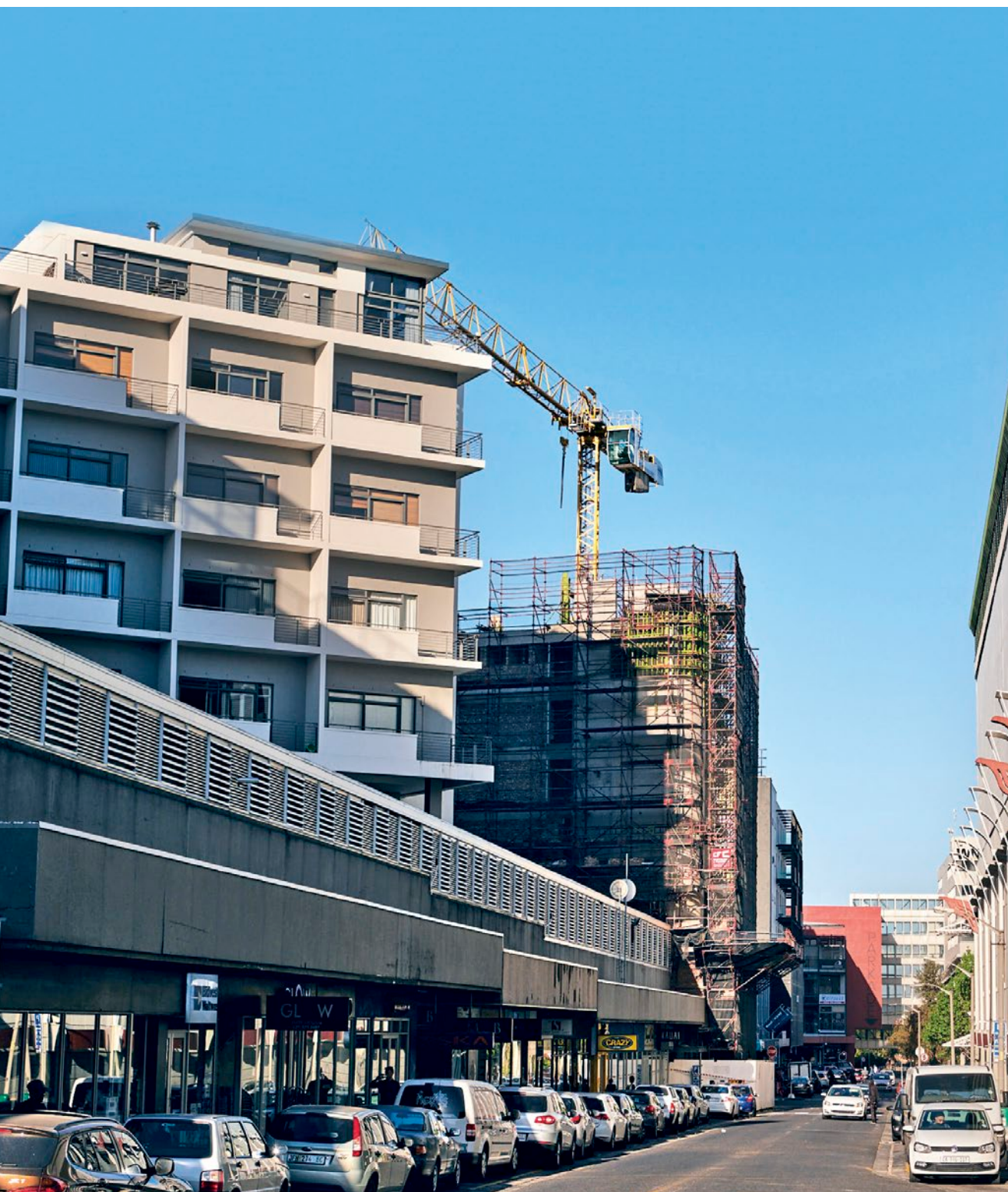
Cavendish and Vineyard Road construction
